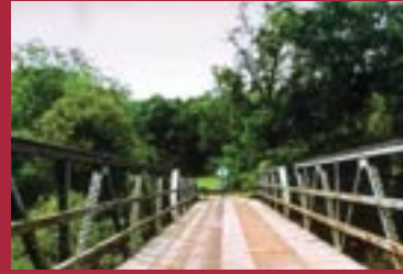
BURROUGHS STREET BRIDGE AND PORTLAND RAILS-TO- TRAILS PORTLAND, MICHIGAN
