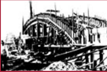
RAINBOW ARCH BRIDGE MORGAN COUNTY, COLORADO
