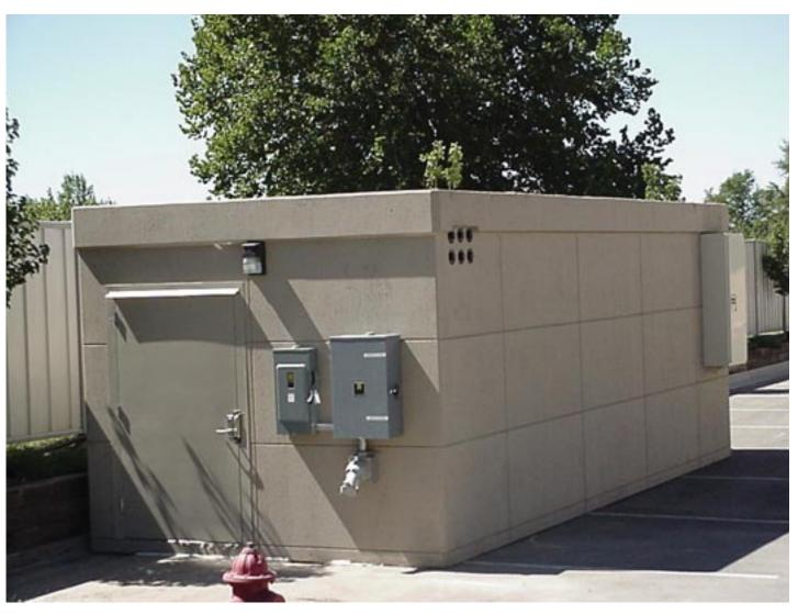
This utility enclosure had to be relocated at the owner's expense. A verbal right of way (a revocable license) was taken by the field engineer and constructed before the right of way agent could make contact with the owner to finalize the easement document. New owners were in possession of the property when the agent contacted them. They had different plans for this parcel and demanded its removal. Total cost of relocation: \$1.14 million.
