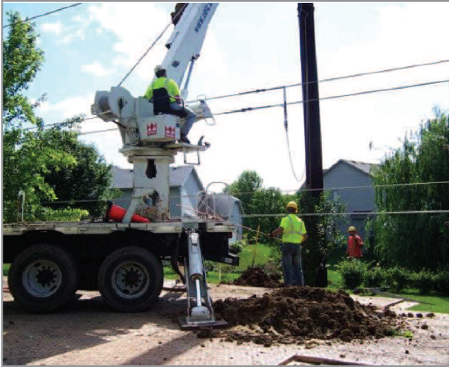
Construction phase of Great River Energy's West Metro 10 mile upgrade.
