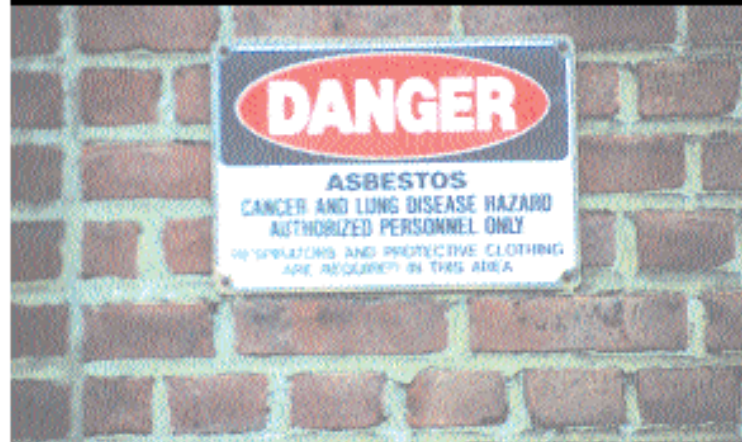
The cost of asbestos abatement at the case study produces a barrier to revitalization. A variance constitutes the only tool that can overcome this impediment.
