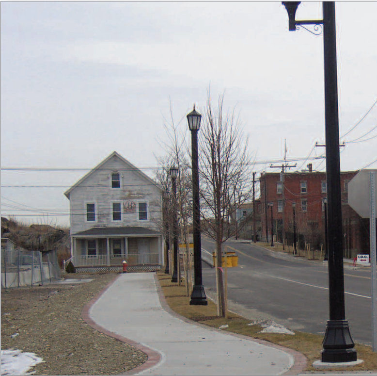
This photo features the house that spilled over onto Walbach Street. This house was a gutted shell several years prior to the Fort Trumbull Project and remained so until demolition in 2007.
