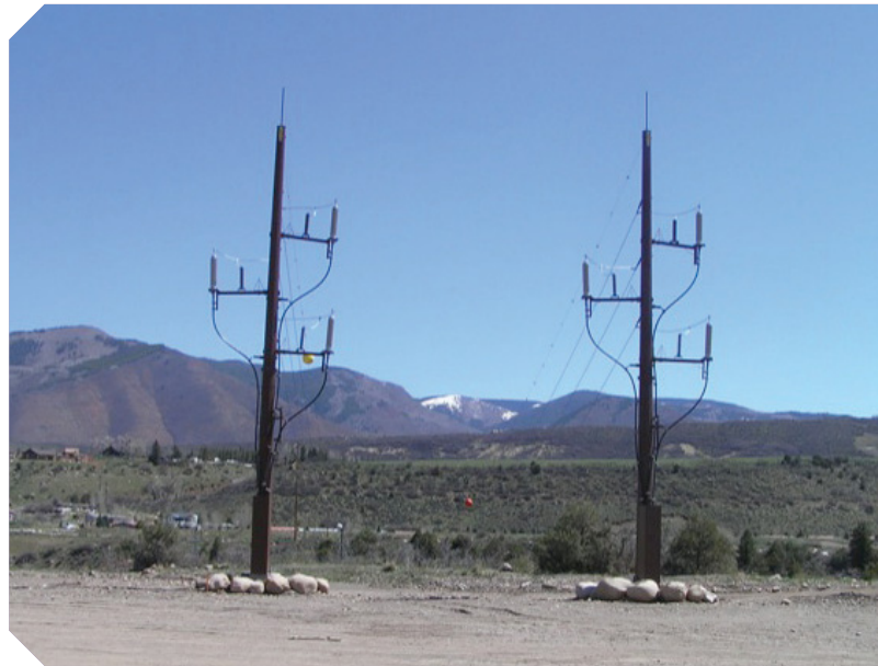
These towers bring the 115 kv line across the Roaring Fork River where it goes immediately under ground to begin its seven-mile journey under Highway 82 to the GIS substation.
