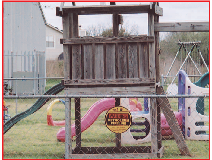
Encroachment issues affecting right of way.
