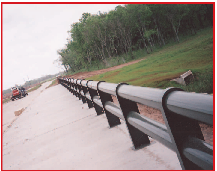
One of many uses for structural pipe is found on this bridge railing.
