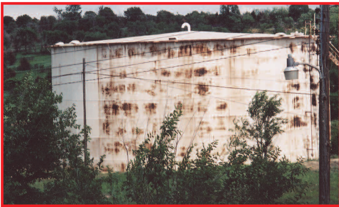
A crude storage tank like this one can be salvaged for plate.
