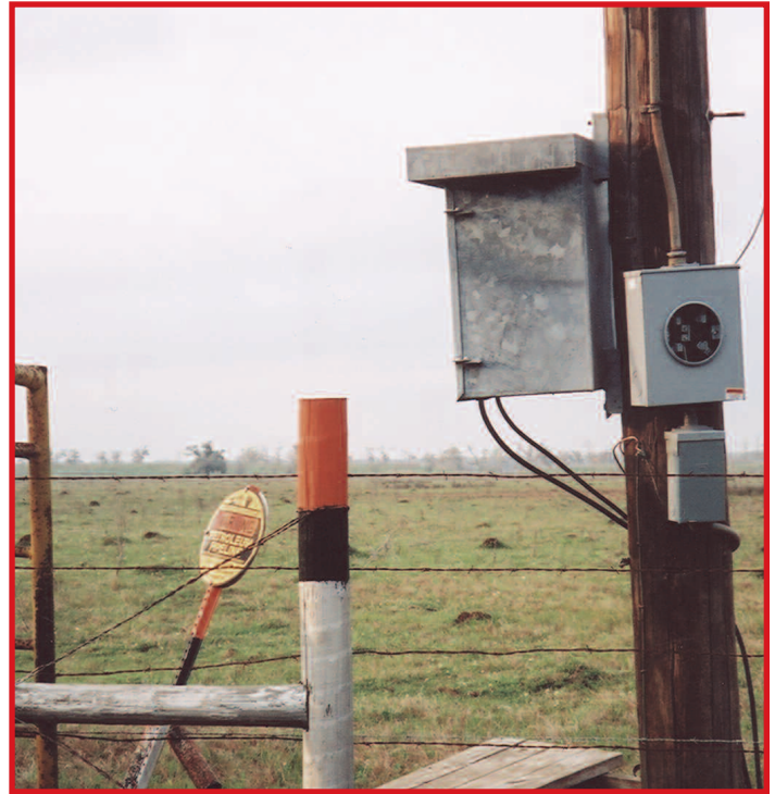
Right of way signage and cathodic protection equipment in despair.
