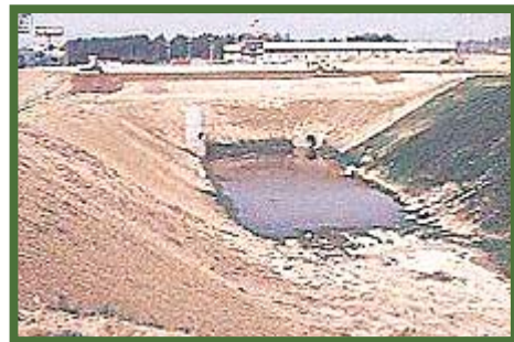
Sediment Pond: A sediment pond is used to capture runoff and allows sediment to settle before water is discharged to storm drains.
