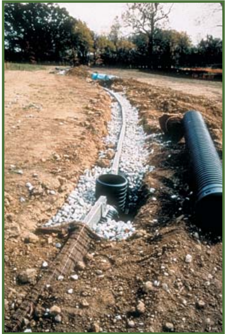
French Drain: This site shows how a french drain can be used to divert storm water or reduce its flow impact on a down slope.
