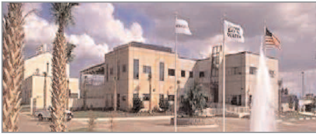
The Surface Water Treatment Plant covers over 200 acres and can produce up to a capacity of 72 mgd. As the cornerstone of the regional system, it treats water from the Alafia and Hillsborough Rivers, the Tampa Bypass Canal and the Reservoir.
