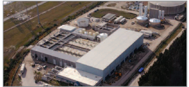
The Seawater Desalination Plant is the largest plant of its kind in North America. A drought-proof component of Tampa Bay Water's drinking water system, it can produce up to 25 mgd and provides six to 10 percent of the region's total drinking water supply.
