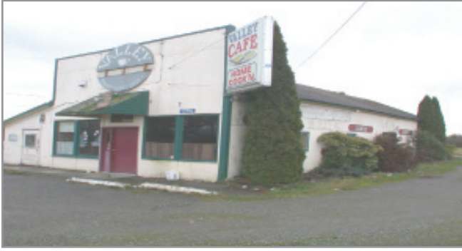
On the northern lot sits the restaurant, septic system with drain field and small parking area.
