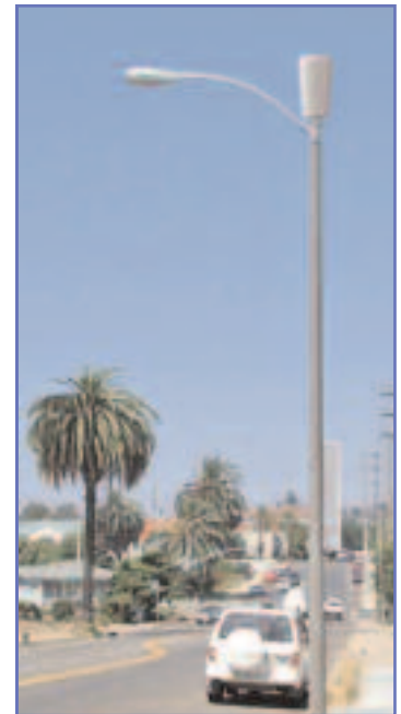
NextG node located midway up pole, over white car (external omni-directional antenna on top)
