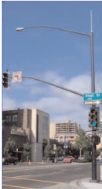
NextG node located inside traffic light (external antenna on top)
