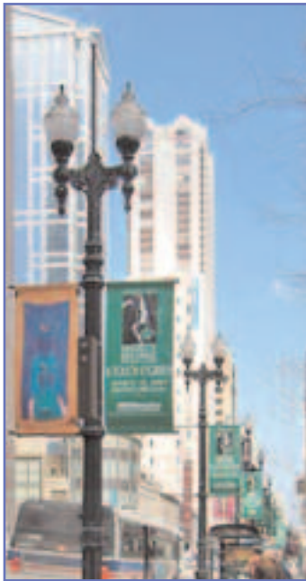
NextG node located on decorative light (between flags) with antenna mounted on top of pole
