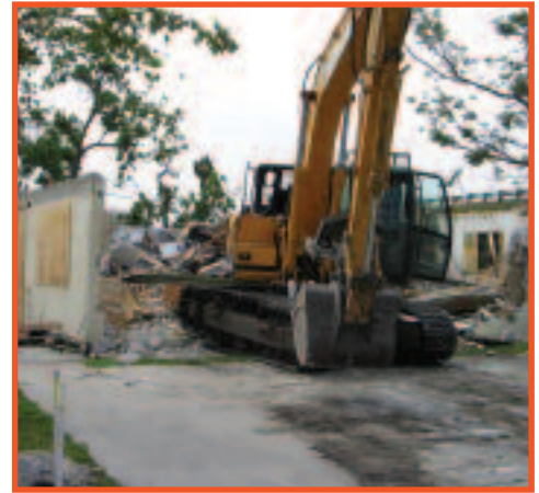
Successful negotiations with homeowners - not auction or condemnation - allowed early acquisition and subsequent demolition of numerous structures.
