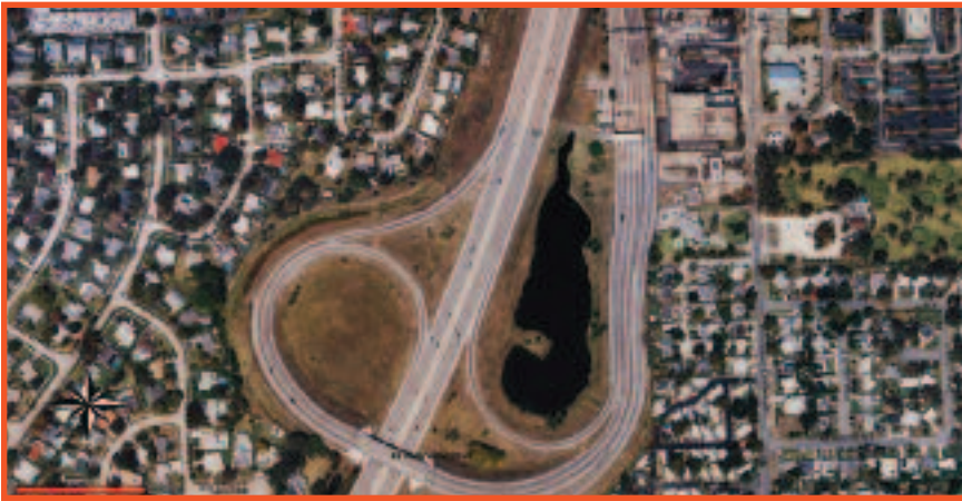
Planned capacity improvements for Hollywood Boulevard Interchange necessitated acquiring of surrounding residential and commercial properties.
