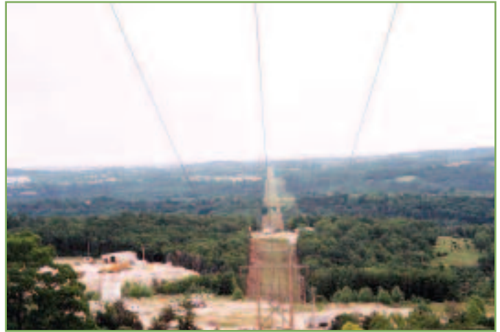
The dipping landscape in Oklahoma shows off one of NRS's well-managed right of ways.
