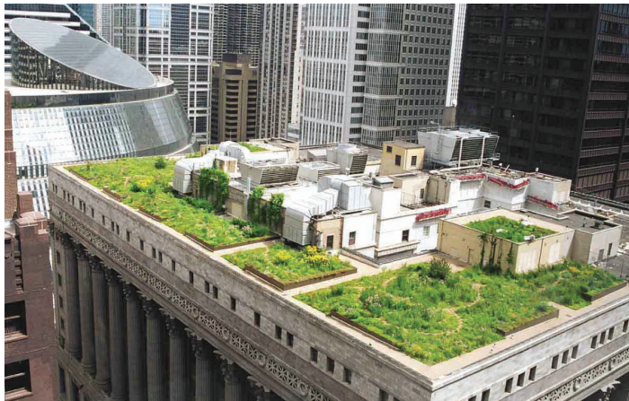
The green roof installed in 2001 on top of Chicago's City Hall reduces water pollution and saves on utility bills.
