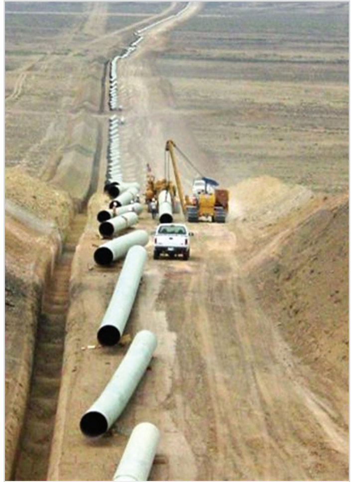
Pipe is laid out along the right of way during REX West construction in Nebraska.
