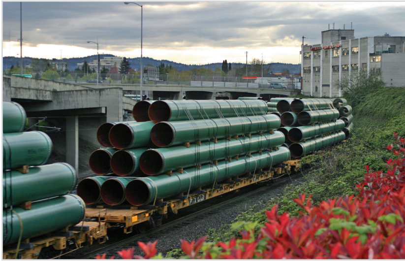
Trains were used to transport pipe throughout REX construction.
