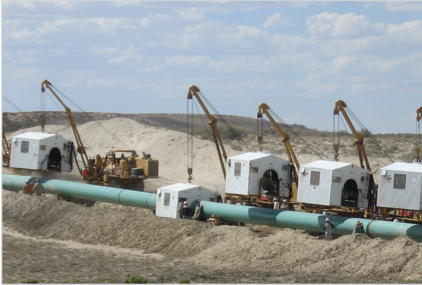
For the mainline construction, pipes were welded using on-site welding shacks.
