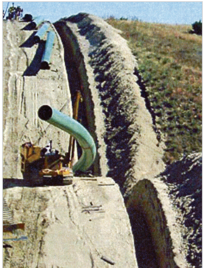
REX West engaged pipe stringing and bending in Wyoming.
