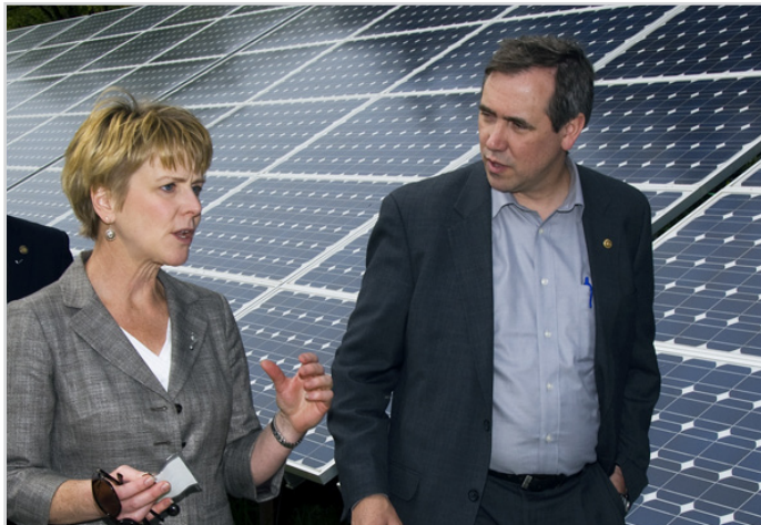
On one of her many site tours, Allison describes to Oregon's U.S. Senator Jeff Merkley how the solar array powers the interchange lighting.
