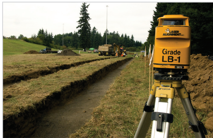
In preparation for solar panel footings, trenching is undertaken in the middle of the intersection.
