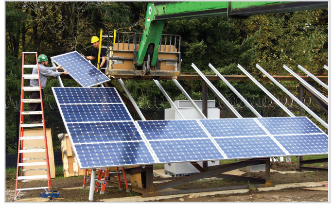
Using the existing right of way, ODOT installs solar panels on the Federally-designated Corridor of the Future.
