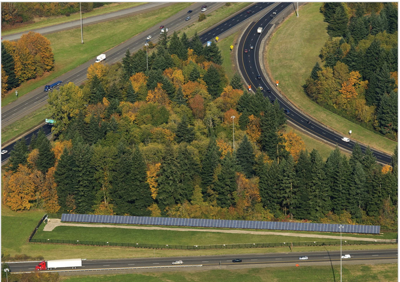
Roughly the size of two football fields, the 104-kilowatt solar photovoltaic system covers 8,000 square feet and connects with the electric power grid on the other side of two major freeways.
