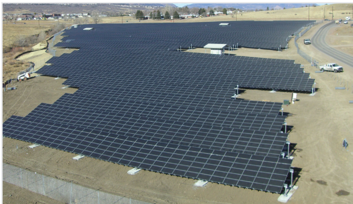
A solar photovoltaic facility now resides at a former landfill site in Fort Carson, CO.
