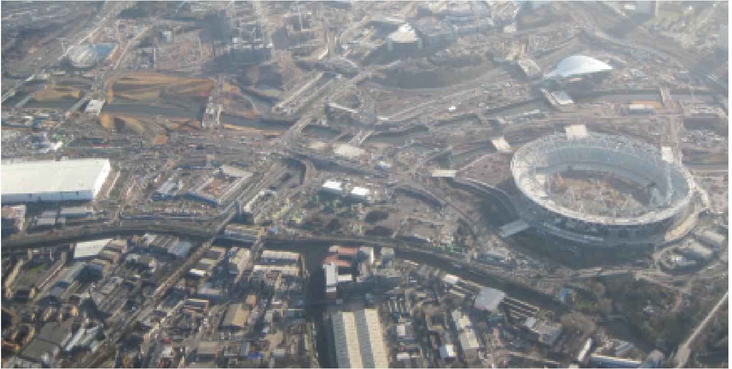
The Olympic zone (looking east) in Spring 2010 shows the main stadium and Aquatics stadium (Wave Roof) on the right, and Media Centre and Velodrome on the left.
