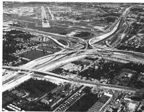
Looking southeast across a major part of the I-595 project nearing completion – the I-595/I-95 four-level interchange and the three-level I-95/S.R. 84 interchange. This $120 million construction contract is DOT's largest ever.
