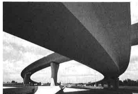
August '89 ground view of nearly completed concrete segmental bridges criss-crossing the interchange.
