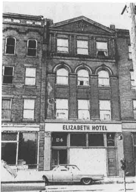
This entire block was demolished to make room for I-279.
