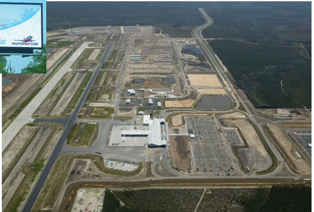
The first new publicly-funded international airport built in the United States since 9/11 has a 10,000-foot primary runway and a LEED certified green building air terminal.
