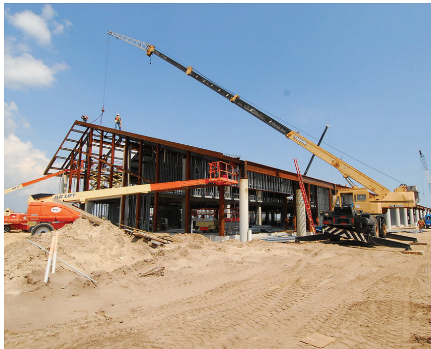
Construction at the new site was well underway when the team was brought in to relocate hundreds of tenants.
