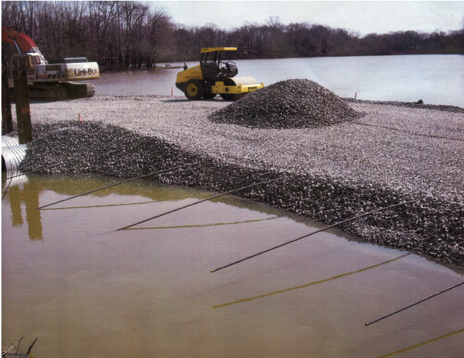
To alleviate potential hardship for the local merchants, a temporary bypass road was built alongside the bridge to maintain traffic flow.
