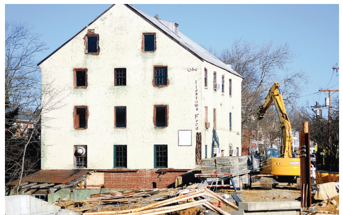
An 18 th century mill building with multi-tenant commercial occupancy required temporary closure during construction.
