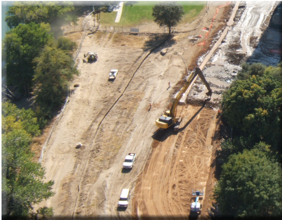
Levee improvements are well underway on the I Street South Levee in the city of West Sacramento.
