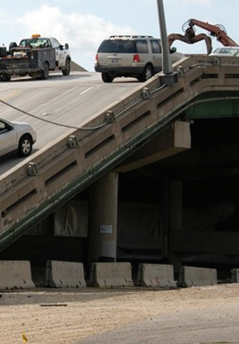
The Minneapolis' I-35W bridge was deemed fracture critical before collapsing in 2007.
