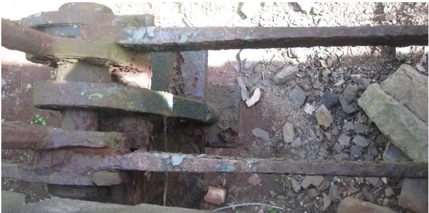
This steel truss bridge, one of the oldest types constructed, was labeled fracture critical like the I-35 bridge, which means if a single tension member fails, the bridge falls.
