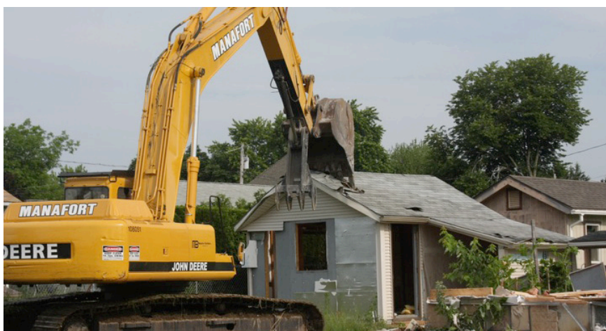
The Greater Springfield Reliability Project required 39 miles of new and reconstructed overhead transmission lines in Connecticut and Massachusetts. Roughly 4,000 abutting properties were impacted.
