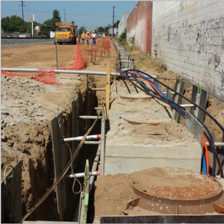
Fiber optic lines are relocated along the railroad right of way in preparation for the installation of a temporary rail detour route.
