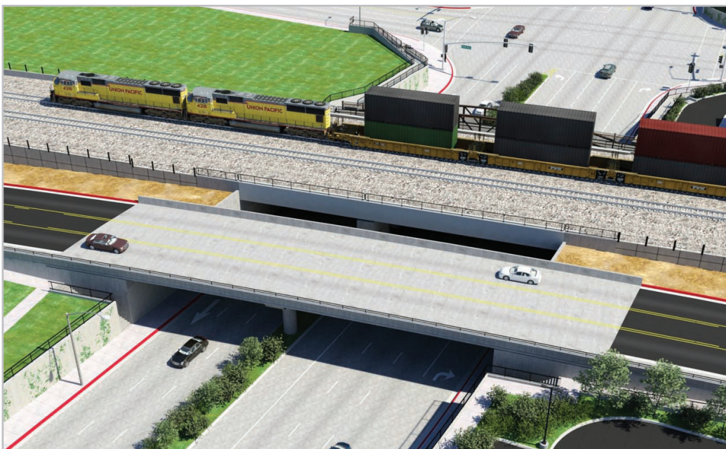
Grade separations, as shown in this computer-generated image, will allow cars to safely cross underneath and over train tracks, reducing accidents, traffic and pollution.
