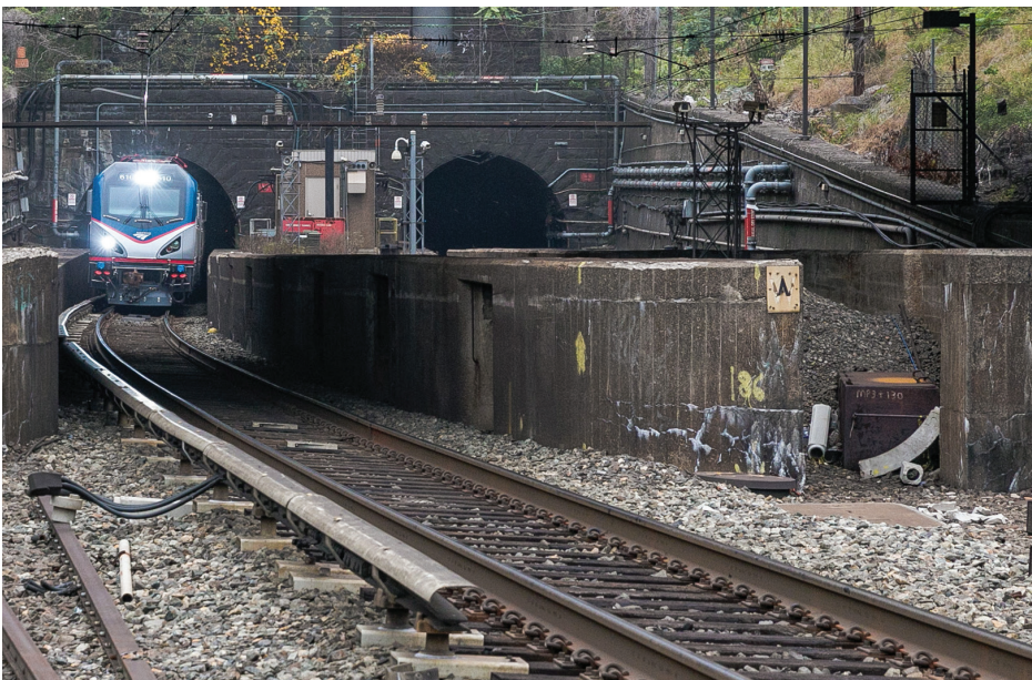
The Gateway Project will expand and renovate the Northeast Corridor rail line between Newark, New Jersey and New York City. The line's original tunnels and bridges were built over 100 years ago and suffered major damage during Hurricane Sandy.
