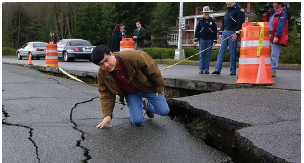
In 2001, then-Washington Governor Gary Locke inspects a roadway after the region survived the strongest earthquake in a half-century. Infrastructure damage was estimated at $2 billion.
