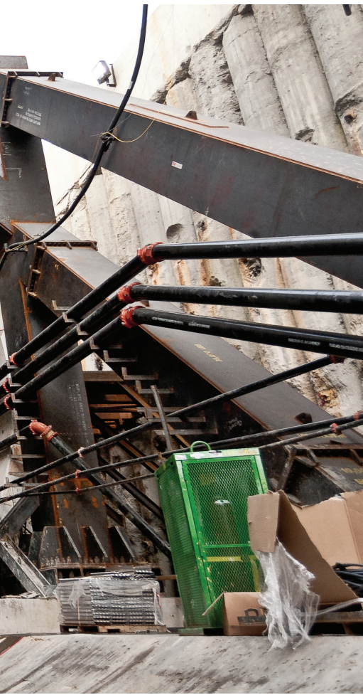
The world's largest diameter bored tunnel beneath downtown Seattle, WA will replace a double-deck highway built in the 1950s, opening to traffic in 2015.
