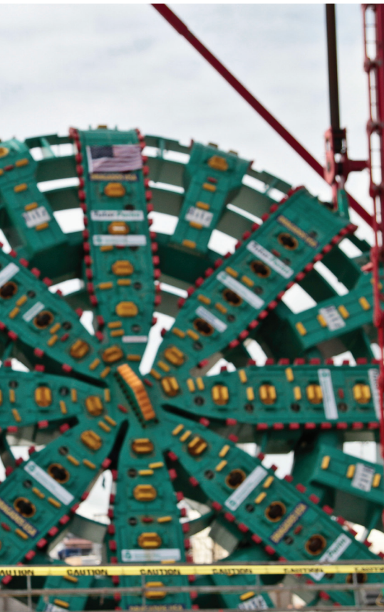
In May 2013, Washington State Secretary of Transportation Lynn Peterson gathered with elected officials as the tunneling machine's five-story-tall cutterhead is lowered into the launch pit.
