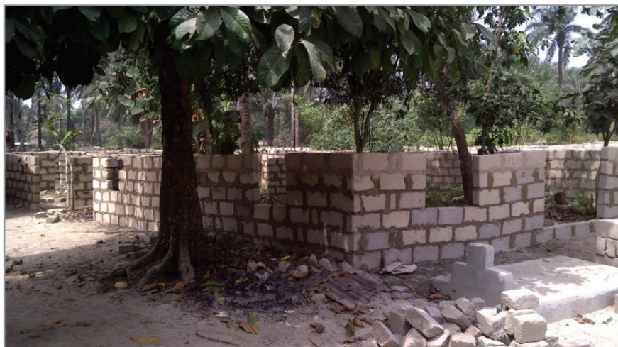
Property acquisition becomes especially challenging when the landowner rushes to build an “emergency” structure in hopes of maximizing their compensation.
