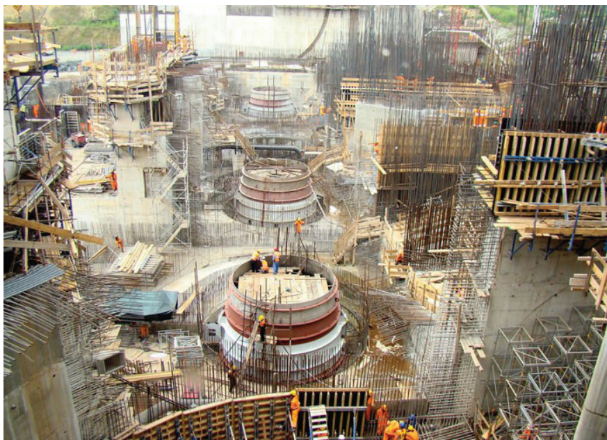
Once completed, Uganda will receive 50 percent of its power from the Karuma hydropower project, a mega-project estimated at $65 million.
