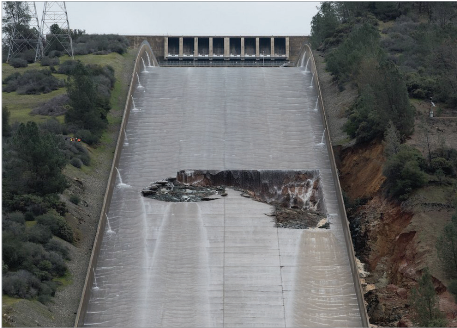
In February 2017, damage to the Oroville Dam's main spillway caused the evacuation of more than 180,000 people living downstream.
