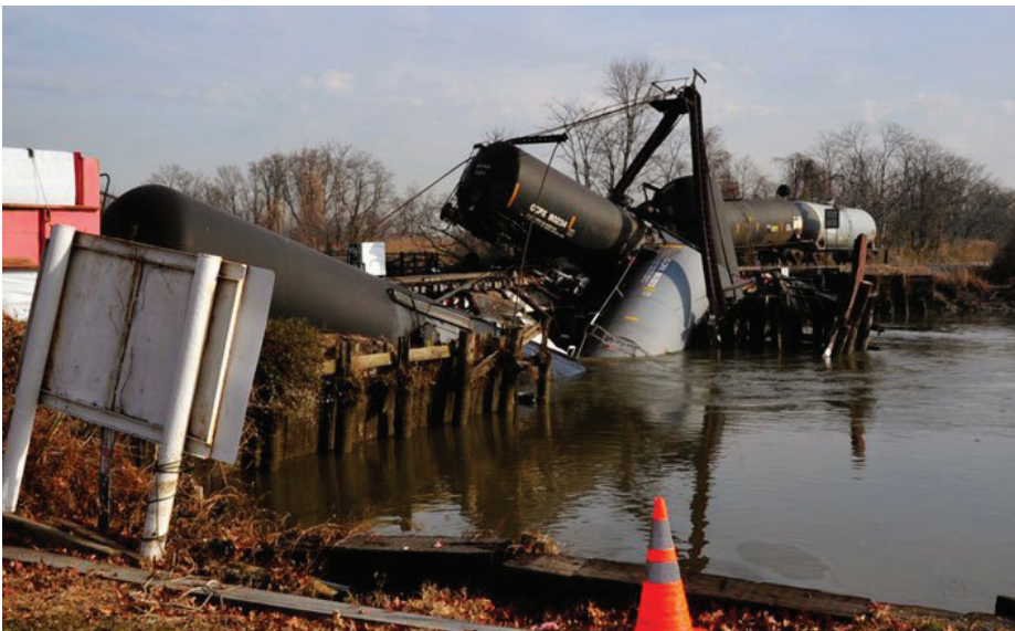
A train reportedly carrying vinyl chloride was derailed in Paulsboro, New Jersey in November 2012 after the railway bridge crossing Mantua Creek collapsed. The derailment prompted a multiagency emergency response.
