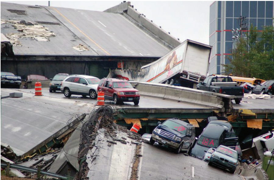
Cars rest on the collapsed portion of the I-35W Mississippi River bridge after the August 2007 collapse in which 13 people were killed and 145 were injured.
