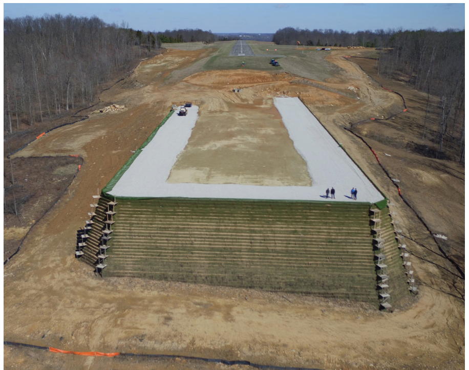
UAS pilots use an unmanned aircraft system to monitor the construction phase of a 500-foot runway extension at the Paoli Municipal Airport in Indiana.
