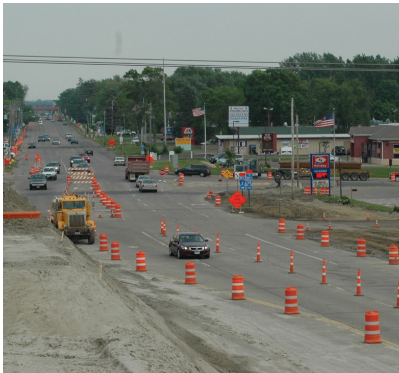
Without skillful utility coordination, utility relocations can cause significant cost increases, street congestion and construction schedule delays.
