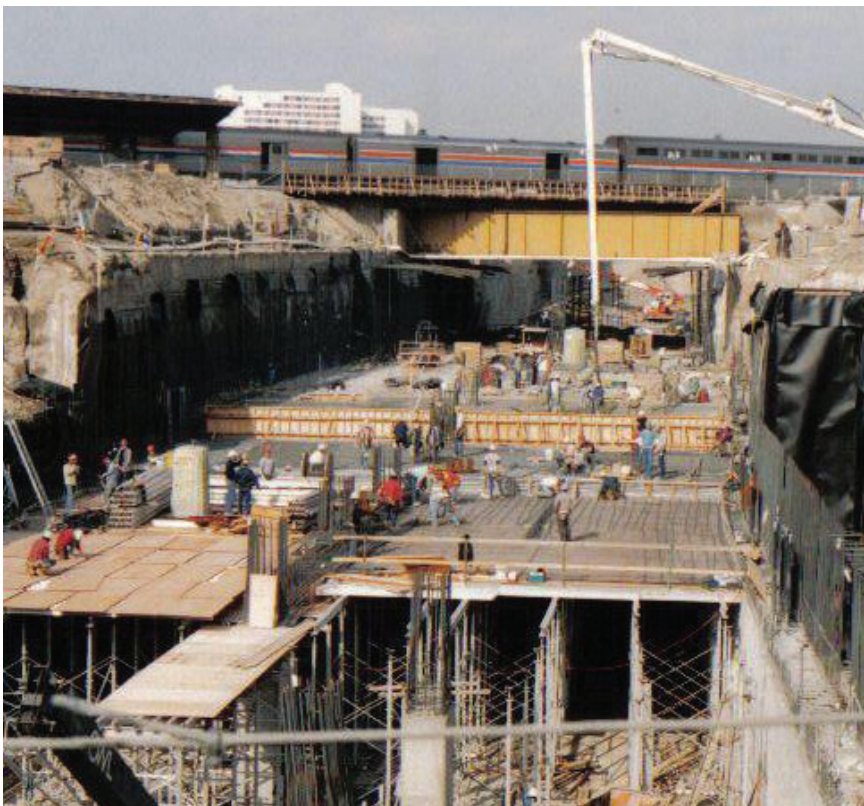
A major metro tunnel project demands coordinating utility relocations with pinpoint scheduling.
