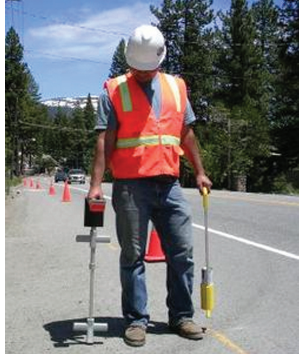
Taking time to accurately locate underground utilities during the planning phase allows minor design adjustments to be made, thereby saving money and preventing unnecessary delays.
