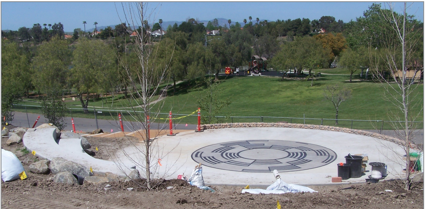
Construction of the outdoor public amphitheater fulfilled a goal set in the park’s 1973 master plan.
