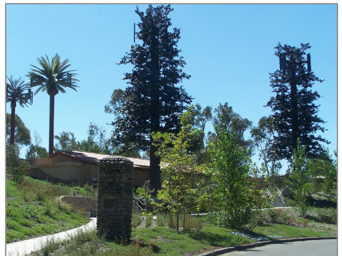
To minimize the visual impact, the 24 antennas were camouflaged within several 60-foot tall faux trees.
