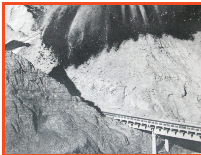
The Division of Highways blasted the slope to make way for the four-lane highway.
