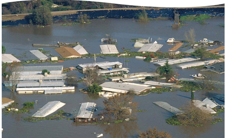
In 1997, a levee break on the Feather River flooded 16,000 acres and forced thousands to flee their homes.
