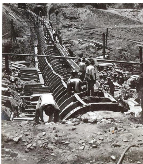
Crews constructing the aqueduct in 1910. Thousands of workers were involved with the project, thanks to high turnover due largely to the harsh living and working conditions that came with the job.
