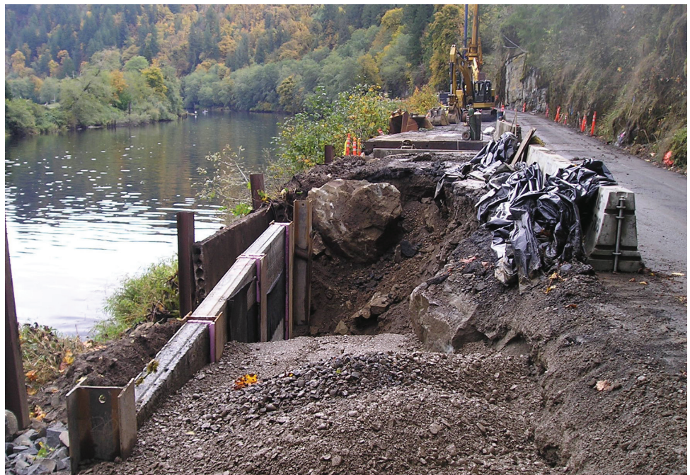
During excavation, construction teams discovered large boulders instead of the expected bedrock.
