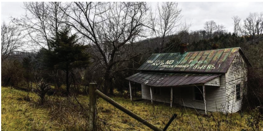
The property owners openly declined survey permission, asserting their right to deny entry.
