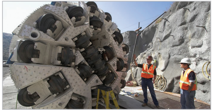
To make way for the San Vicente Pipeline tunnel, an 11.5-foot hard rock boring machine was used to penetrate 5,255 feet of granitic rocks.
