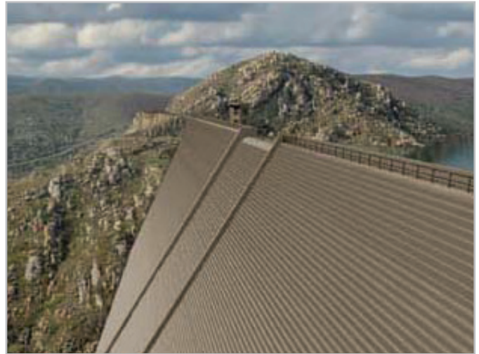
Scheduled for completion in 2014, the San Vicente Dam raise will nearly triple the current water capacity.
