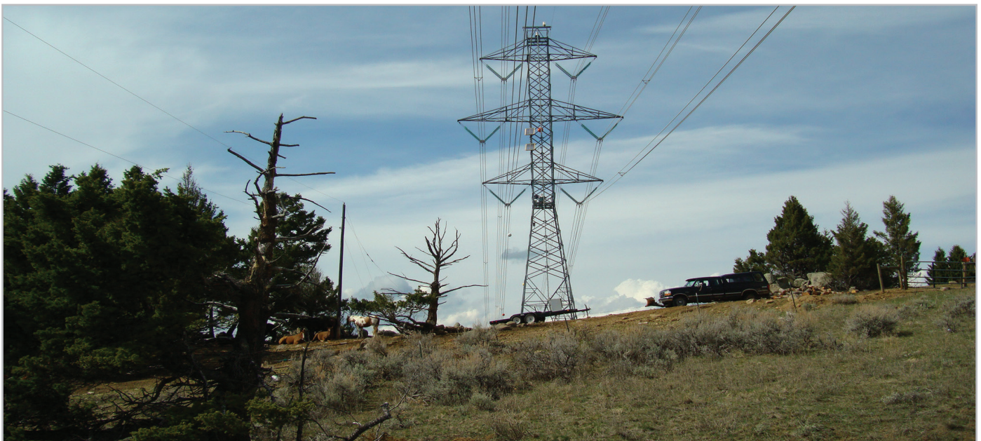
At the time lot sales began in 1986, the transmission lines were already in place.
