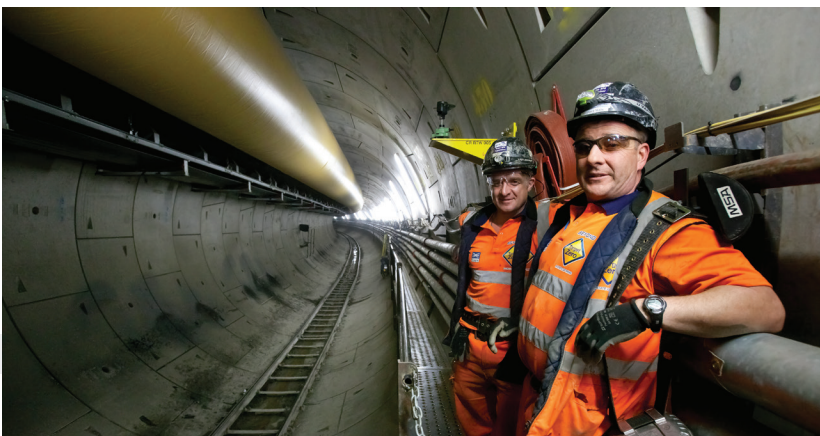
Workers in the Western tunnels of the Elizabeth line.
