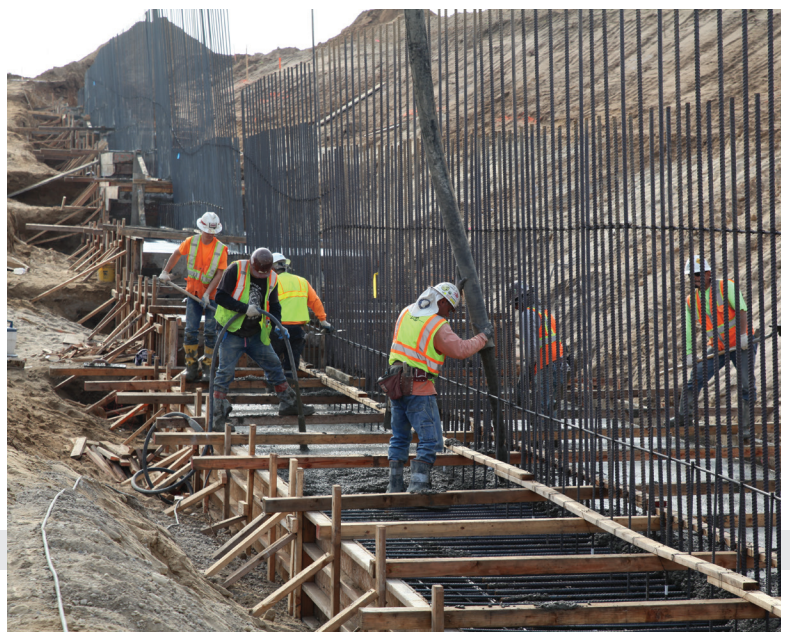
Realignment project in Fresno, California to make way for the high-speed rail line.
