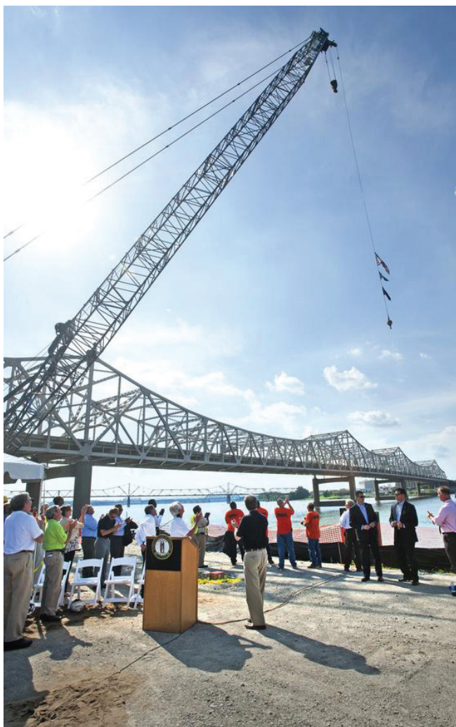
During a recent groundbreaking ceremony, a crane hoisted the American, Kentucky and Indiana flags over a construction site for the downtown span of the Ohio River Bridges Project.
