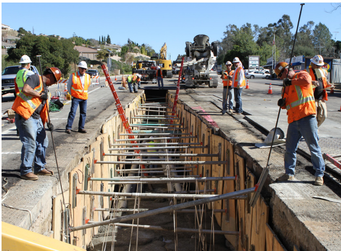
Roughly six miles had to be built beneath Alpine Boulevard, the main county road, so SDG&E constructed streetscape improvements to mitigate the inconvenience to the community.
