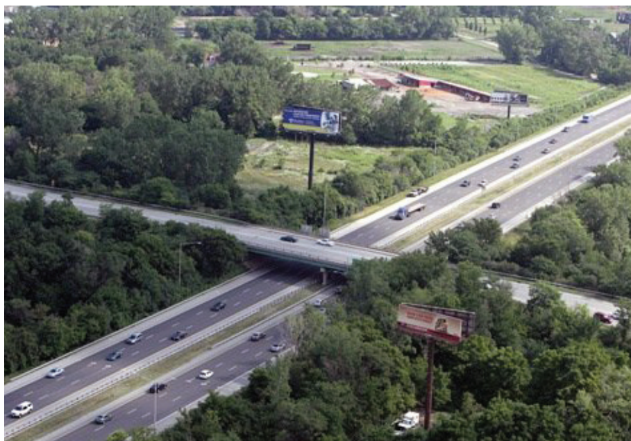
For more than 50 years, the I-294 and I-57 crossed in the south side of the Chicago metro area, but never connected.
