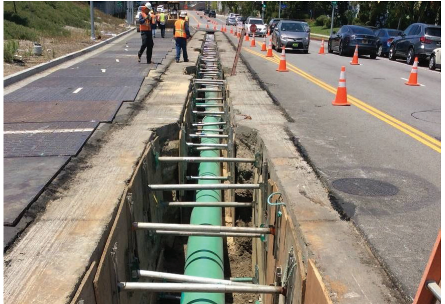
SoCalGas crews work on Line 43-121 North Section 2 in Los Angeles, California.
