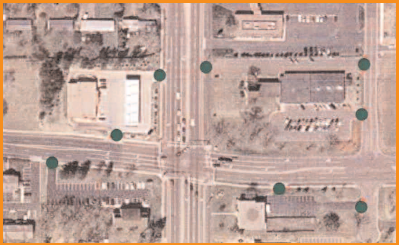
Example #2: Properties on streets with medians develop alternative access points to address one direction front access.
