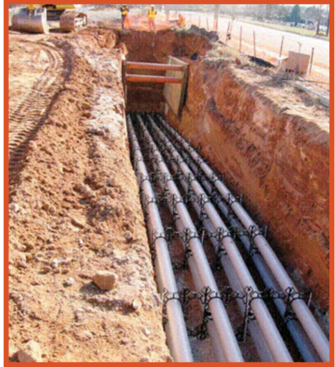
Underground projects prove far more complex throughout each phase.
