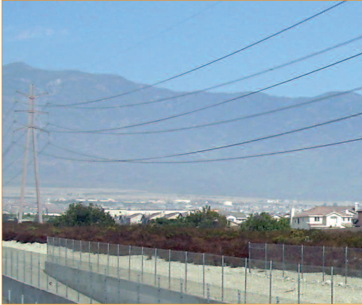
Southern California Edison right of way in Rancho Cucamonga, CA
