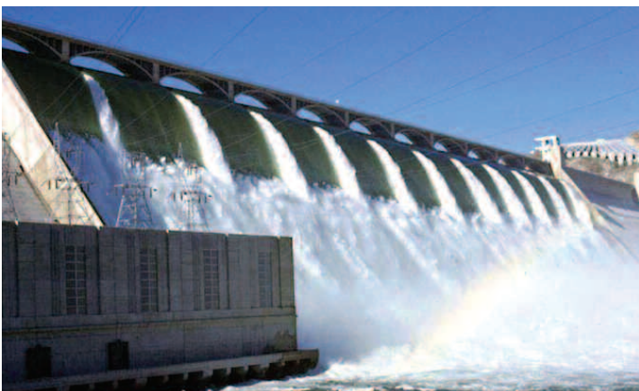
Spillways at Grand Coulee Dam on the Columbia River in Washington. Grand Coulee was designed so that after passing through the power plants at peak hours, water can be pumped back up into the reservoir during non-peak hours for use at the next peaking period.
