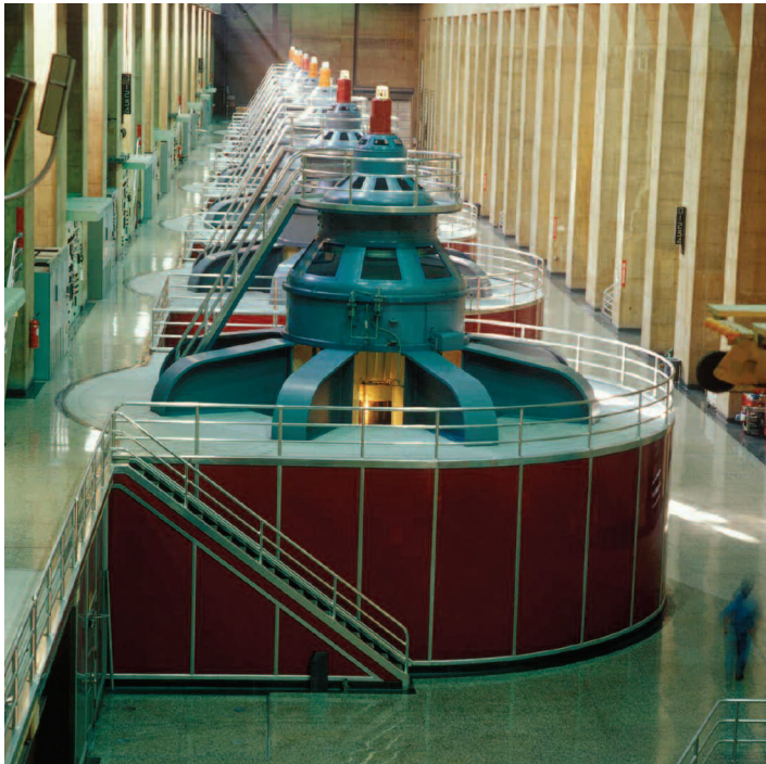
Generators in the Nevada power plant at Hoover Dam. Another similar powerplant is on the Arizona side. Hoover Dam's powerplants generate over 3 billion kilowatthours of electricity annually.
